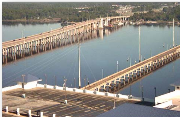
Biloxi, Back Bay Bascule Bridge (MDOT US 1-110)
